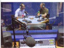
The facility is fully equipped for most forms of radio broadcasts. It is built around a Sonifex S2-15 desk and custom-made furniture. Munro Acoustics managed acoustic design of the studios. Connectivity to the outside world is via Telos Zephyr Xstream ISDN codecs and Sonifex HY03 telephone hybrids. Genelec 8030 loudspeakers and beyerdynamic headphones and microphones round out the kit.
